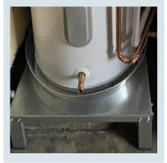
Install a drain pan if there is a wooden floor or if the tank utilizes leak detection.
