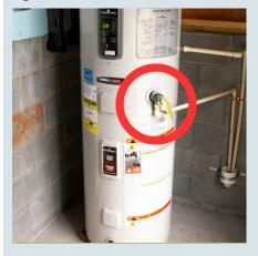
Ensure the pipe terminates according to code.
