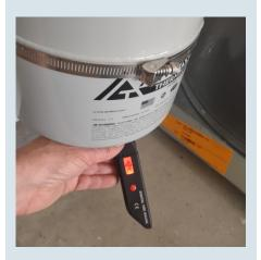
Shut off water and power to the unit. Confirm the power is off with a voltage tester.
