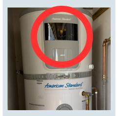
Ensure easy access to drain the tank.
