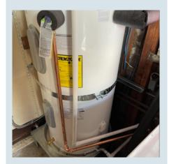
Connect the T&P discharge pipe. Consider using a plastic pipe, if allowable by code.
