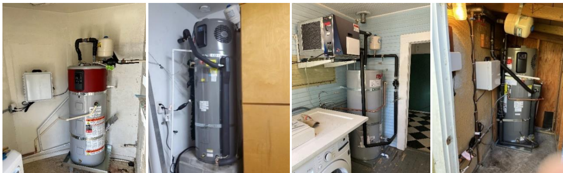
FIGURE 1. EXAMPLE 120-VOLT HPWH INSTALLATIONS
