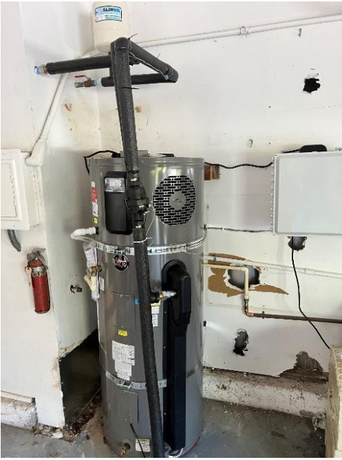
FIGURE 41. IMAGE SHOWING TEMPERATURE SENSOR AT COLD WATER INLET
