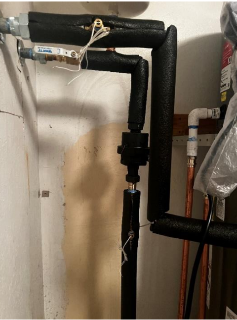
FIGURE 41. IMAGE SHOWING TEMPERATURE SENSOR AT COLD WATER INLET
