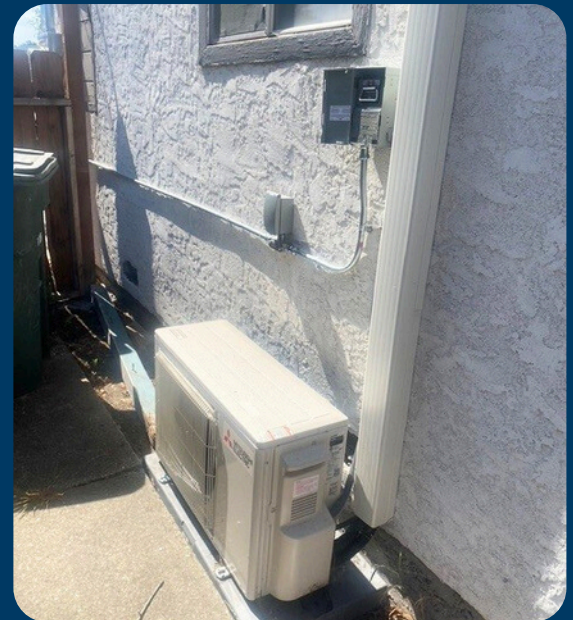
Figure 1: Typical Retrofit Condenser Installation
